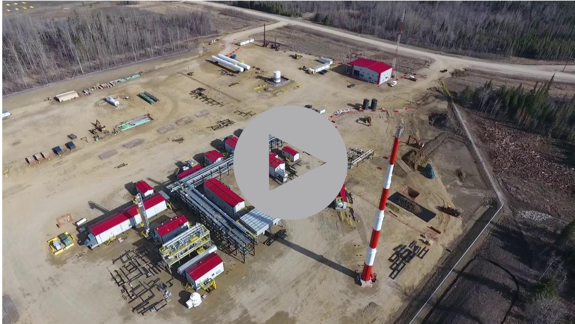
Aerial footage of Pembina's HVP growth projects
